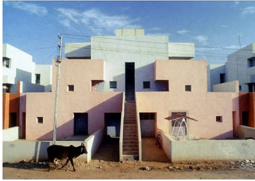
House in its original configuration before the residents move in: Housing for Life Insurance Corporation (LIC), Ahmedabad, 1973 © Vastushilpa Foundation, Ahmedabad
